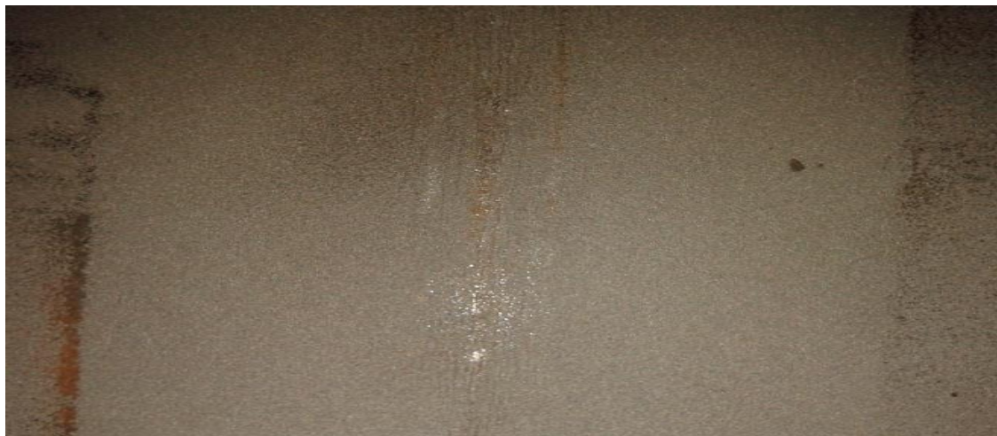
Fig.12 Crack initiation after Bend test
